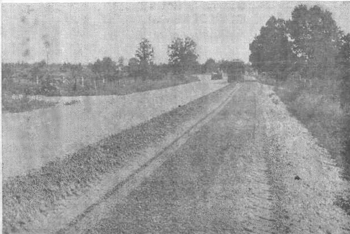
EASTPORT ROAD PAVING UNDERWAY —Work has begun on paving the Eastport Road between Iuka and Eastport. Here machinery is shown preparing the roadbed for the first layer of bituminous prime. When finished the road will have a double bituminous surface and will be a real improvement in the county road system. This section of road is adjacent to Toe Nail Cemetery.
