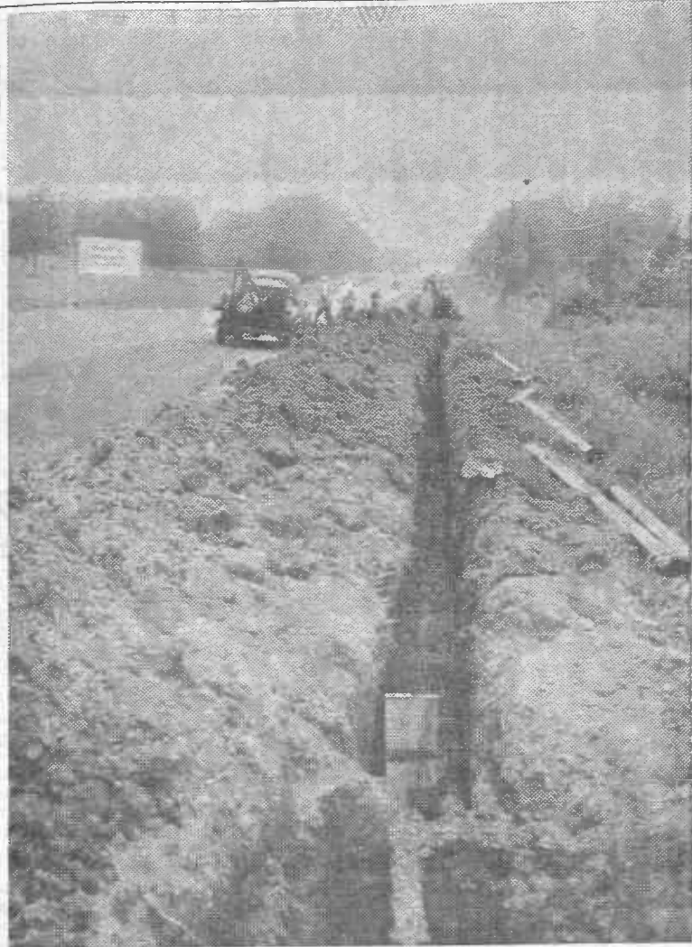
WATER LINE CONSTRUCTION BEGINS —Installation of the municipal water line extensions got underway last week. Here workmen are shown as they began ditching operations along Highway 72-W just beyond the entrance to Tishomingo County Hospital. The remaining extensions of the entire system are expected to be completed in September.
